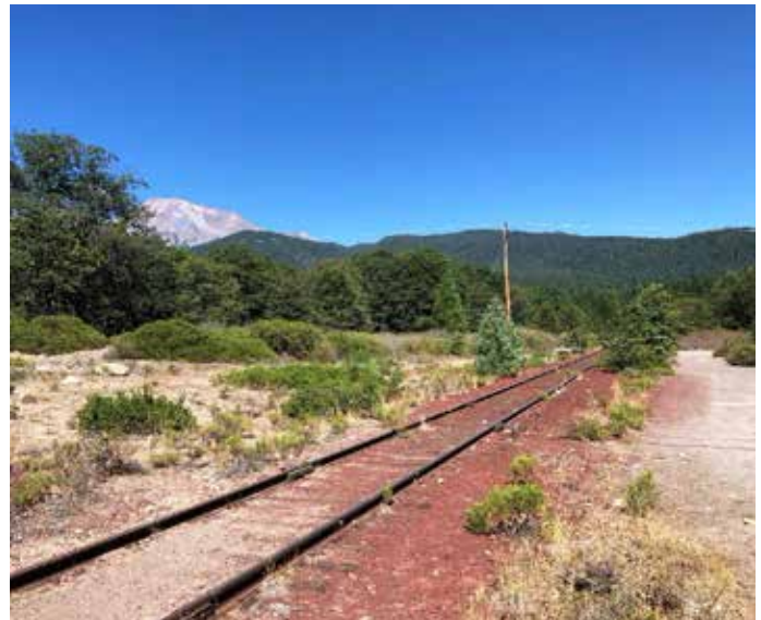
McCloud River Railroad tracks.
